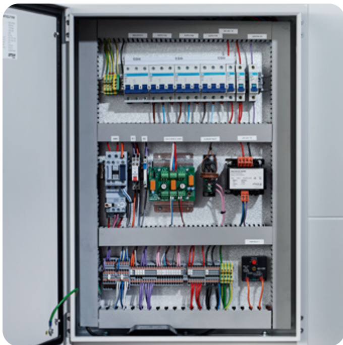
Typical electrical board
