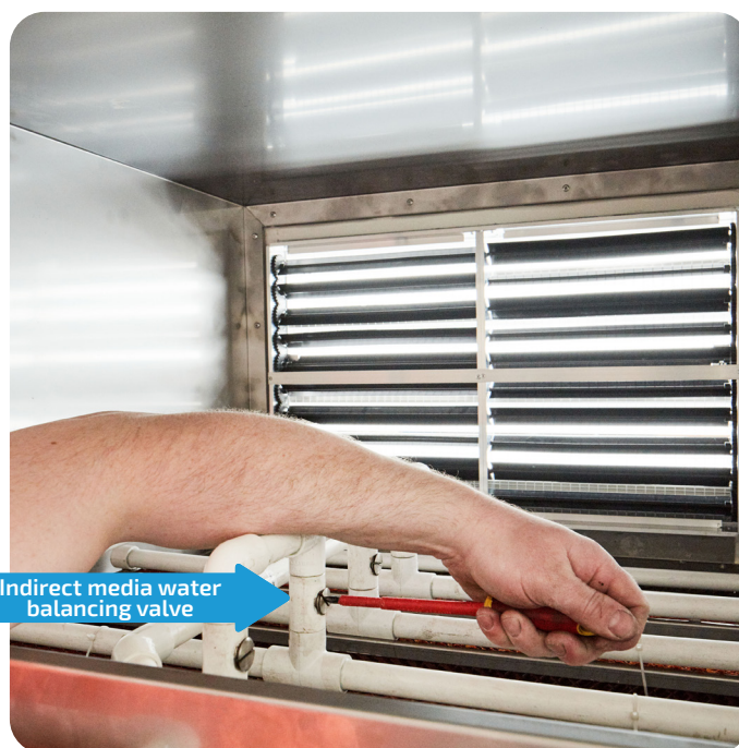
Manual balancing of water flow
