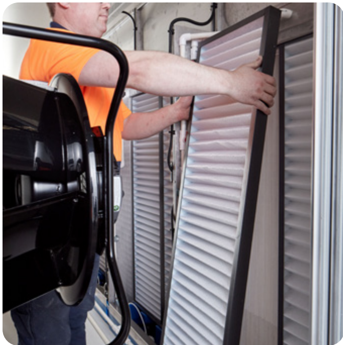
Filter removal and cleaning
