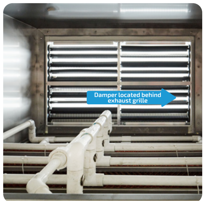
Damper located behind exhaust grille
